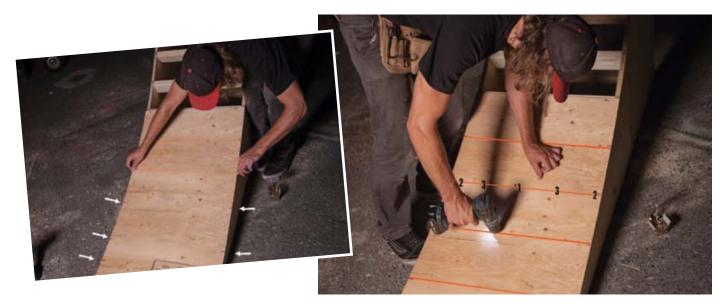
Add screws in all ribs, first in the centre, then one on either outside edge, then add screws in between each of the previous screws. This will help prevent warping.
