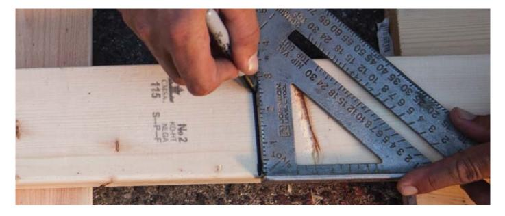
Before you cut your ribs, double check your rib measurements. If they are correct, place 2 of your scrap 2x4s underneath to lift the wood you will be cutting off of the ground. Make sure your supporting 2x4 or work surface is not going to interfere with the saw when it passes over your cut line.
