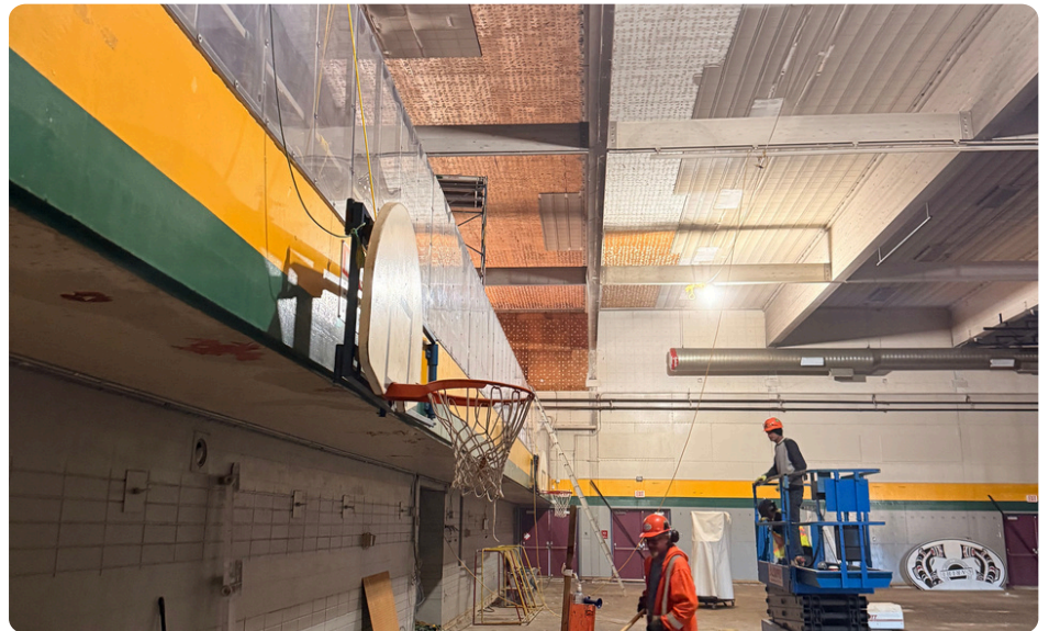
Above: Crews removing the acoustic panels from the ceiling above the gym.
